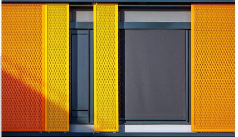
Over 640 cabled motorised roller blinds from ATES, made with Mermet's Satiné 5500 fabric in colour 3030 Charcoal were installed externally. These vertical blinds are able to:
